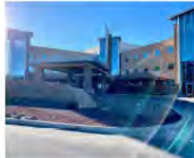
Canyon Vista Medical Center
